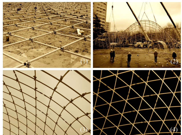
Fig. 6. Assembly (1) | Erection (2) | Erected grid (3) | Braced grid (4)
