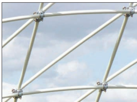
Fig. 14: Meshes before bracing (left). Mesh after bracing (right)
