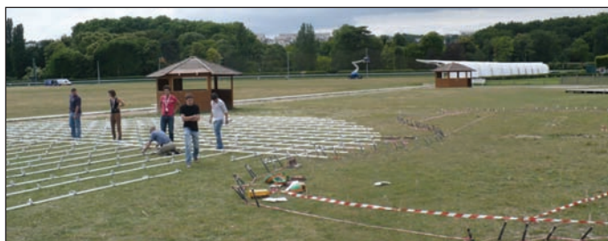
Fig. 11: Initial grid assembled next to the final place of the gridshell
