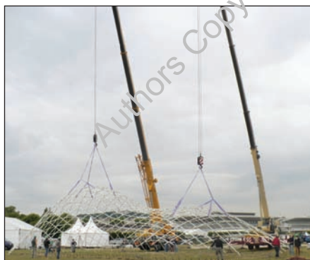
Fig. 13: Lifting of the prototypes by the two cranes
