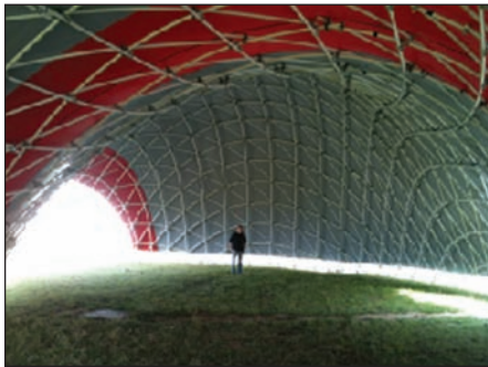
Fig. 18: Inside view of the gridshell
