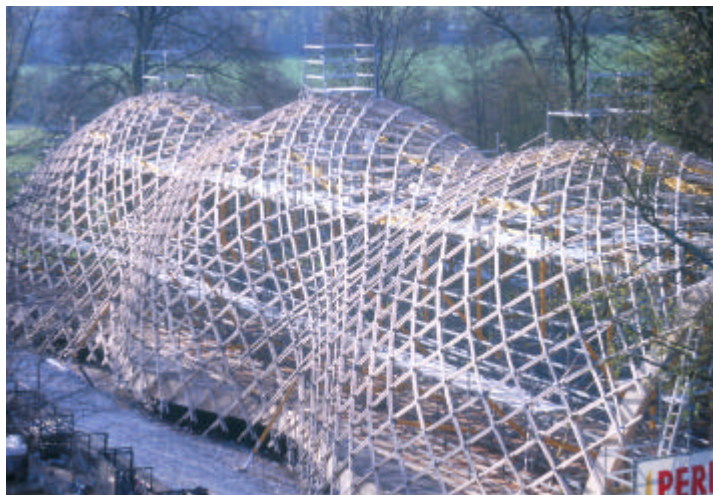
Figure 4.22: Final Shape from East Scaffold Tower
