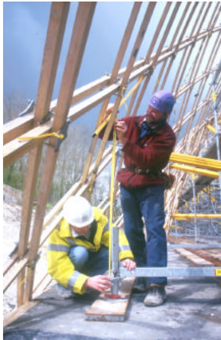
Figure 4.19: Measuring the Gridshell with a Plum-line
