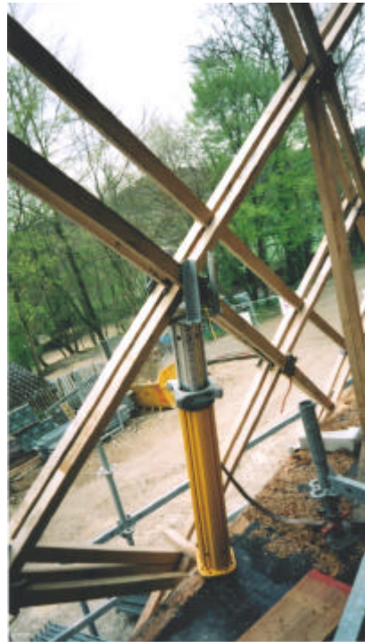
Figure 4.20: Small MULTIPROP pushing up Perimeter Node
