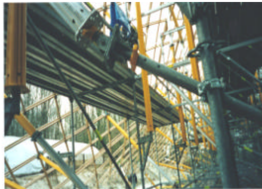
Figure 4.18: Universal Joint at base of Raking MULTIPROP
