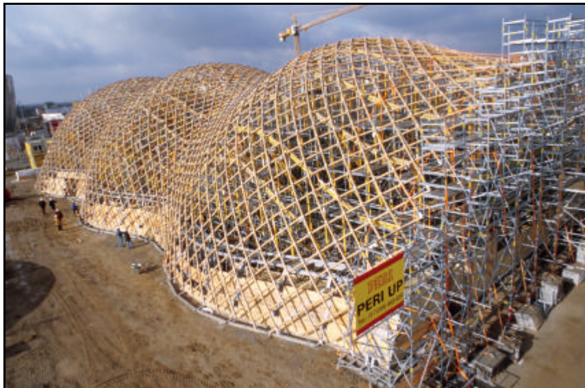
Figure 3.4: Erection of Hanover Gridshell using PERI Scaffolding.
