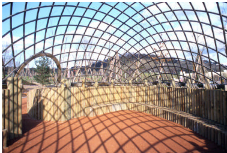
Figure 3.2: The Gridshell at the Earth Centre in Doncaster
