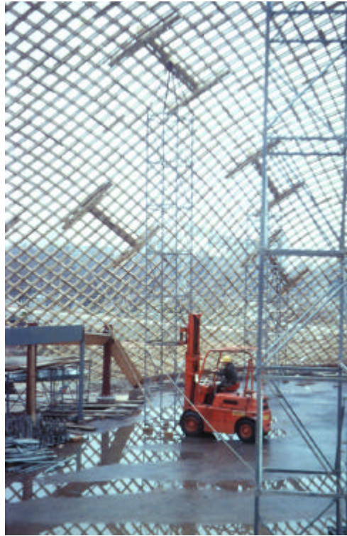
Figure 3.1: Construction of the Mannheim Gridshell
