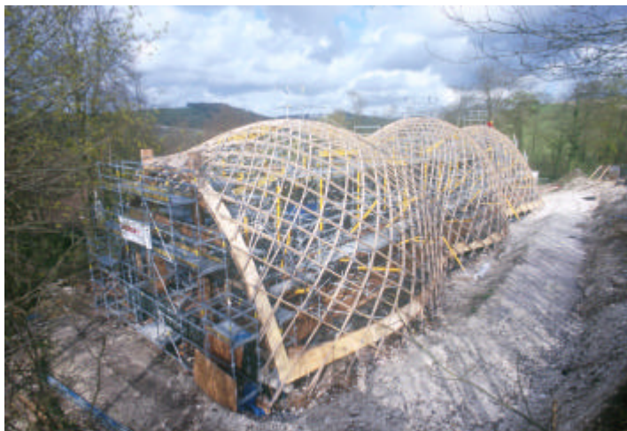
Figure 4.23: Final Shape from West Platform
