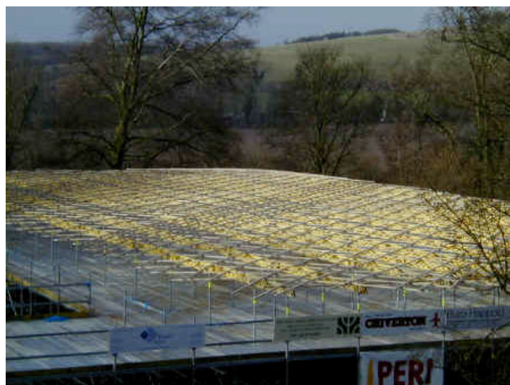
Figure 4.3: The Completed Layout of the Flat Lattice Mat
