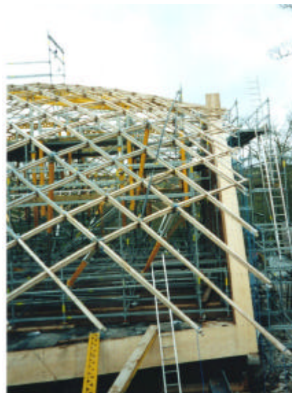
Figure 4.14: Photograph of Gable End Strapping System
