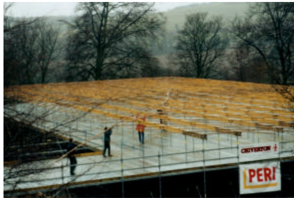
Figure 4.6: Carrying Laths on Scaffolding Platform
