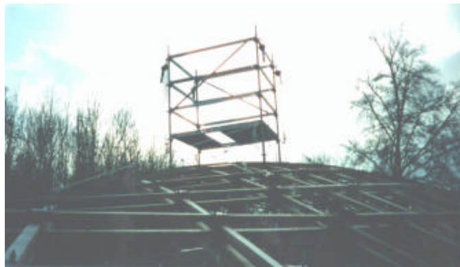
Figure 4.16: Winch System for Centre Crown
