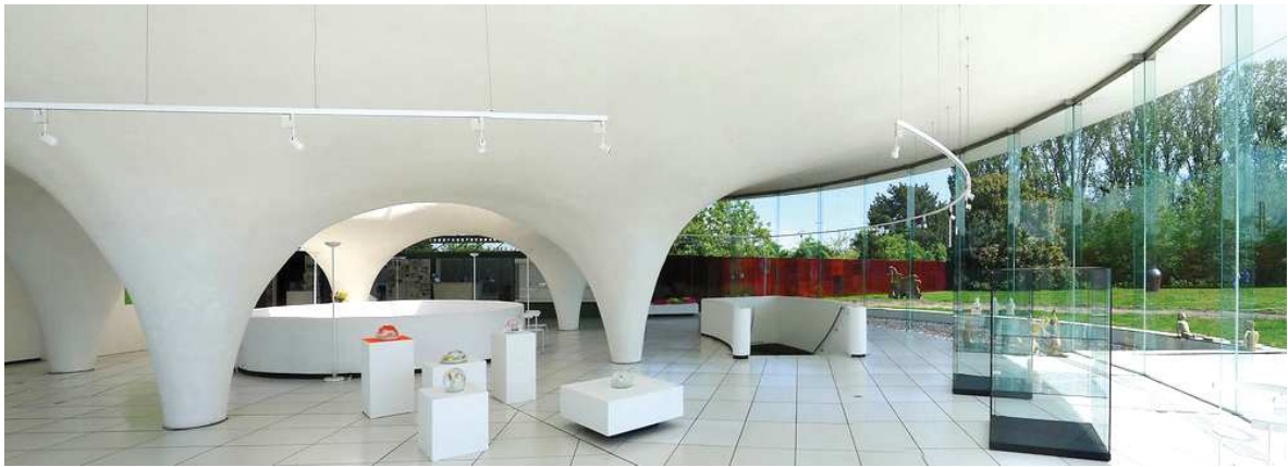
Figure 4: The concrete shell of the Keramion museum in Frechen, Germany, is a Pelikan surface – a special type of i-liwein surface also referred to as i-minimal ©Klaas Vermaas.
