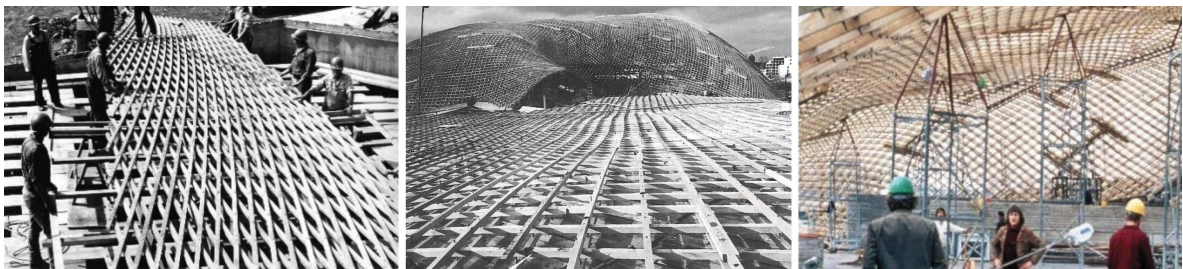
Figure 1: Multihalle in Mannheim: Application of elastic grid deformation (erection). The final shape is determined by scaffolding, without directed deformation behaviour.
