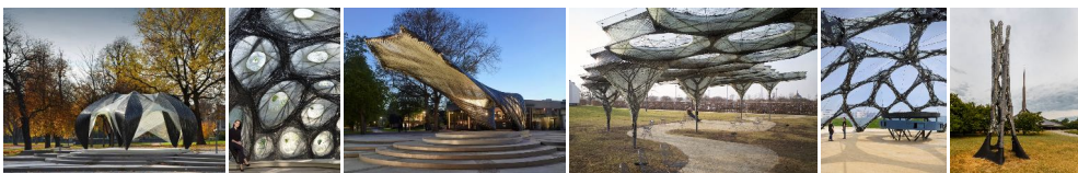
Figure 1: Previous work on load-bearing structures realized in coreless filament winding. (a) ICD/ITKE Research Pavilion 2012, (b) ICD/ITKE Research Pavilion 2013-14, (c) ICD/ITKE Research Pavilion 2016-17, (d) Elytra Pavilion 2016, (e) BUGA Fibre Pavilion 2019 [itke.uni-stuttgart.de], (f) Marshall Prado, UTK Filament Tower 2019 [Hadley Fruits].
