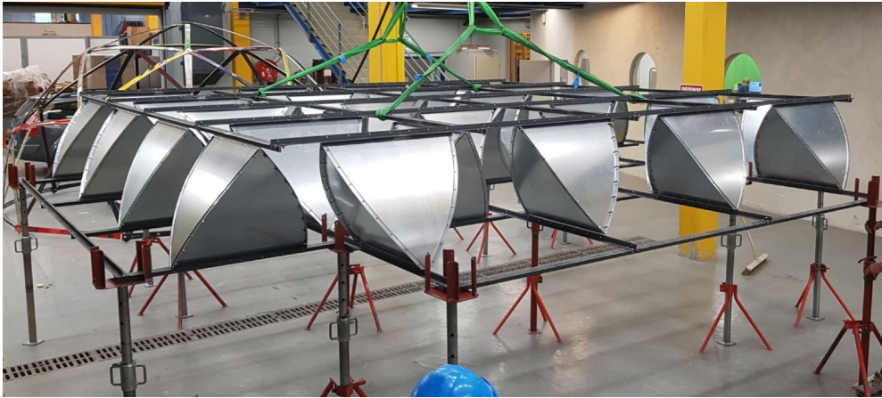
Figure 1: Full scale prototype exhibiting closed piecewise developable surfaces acting as shear components in a double-layer space structure.
